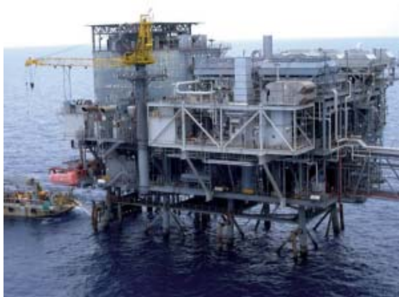
This platform in the Natuna Sea uses CO 2 suppression on its Avon compression package
